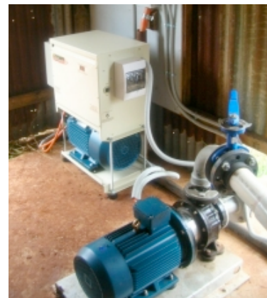
An 8kw 3-Phase Power Converter operating an irrigation pump
